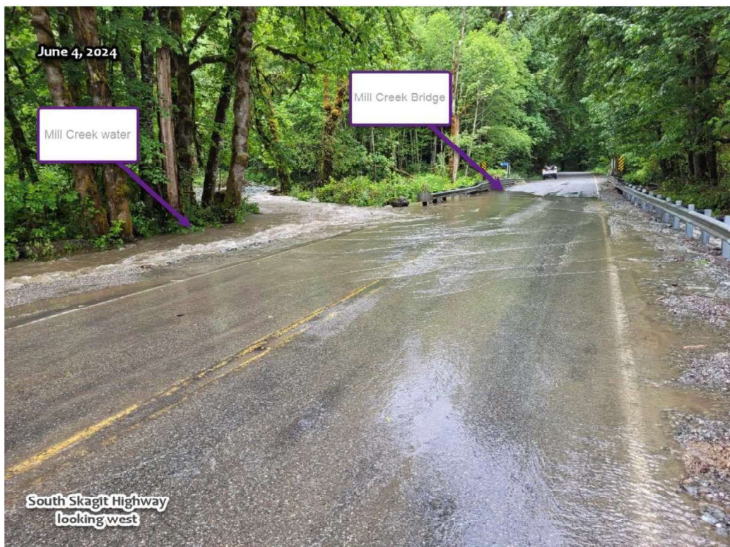
South Skagit Highway looking west on June 4, 2024, same day as above. The majority of Mill Creek is flowing along the highway and into Savage Creek.
