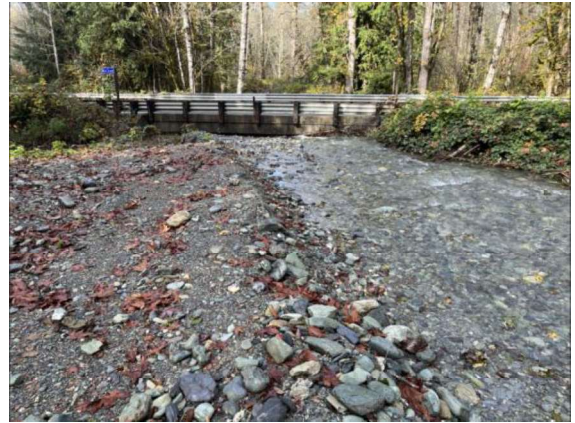
Mill Creek bridge. Picture on the left shows over 50% of the creek avulsing east towards Savage Creek. Picture on the right shows the mostly plugged bridge. This is despite routine dredging. Photos taken October 2024.
