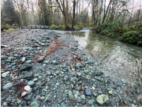
Mill Creek bridge. Picture on the left shows over 50% of the creek avulsing east towards Savage Creek. Picture on the right shows the mostly plugged bridge. This is despite routine dredging. Photos taken October 2024.
