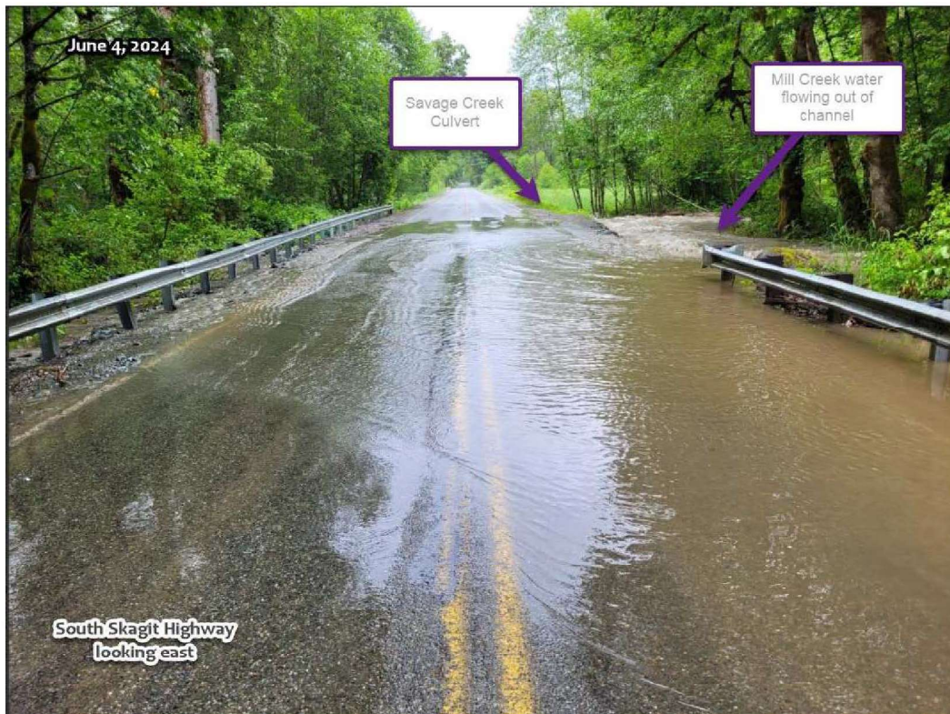
South Skagit Highway looking east on June 4, 2024. A small rain event caused Mill Creek to overtop the road, causing road shoulder damage, impacting drivers, and impacting fish.
